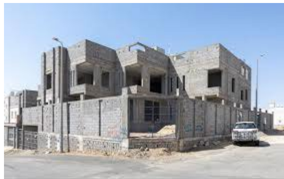
Figure (8): Depicts A picture of a building in Taif made of concrete blocks.
