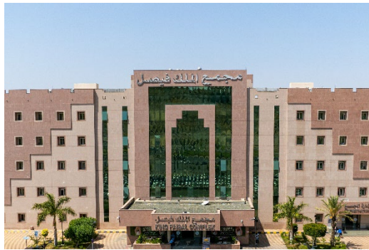
Figure (3): A picture of King Faisal Hospital, whose facades were covered with natural granite.
