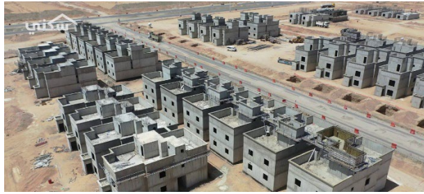
Figure (7): Depicts the application of reinforced concrete in the walls and ceilings of villas in Al-Ward City, Taif.
