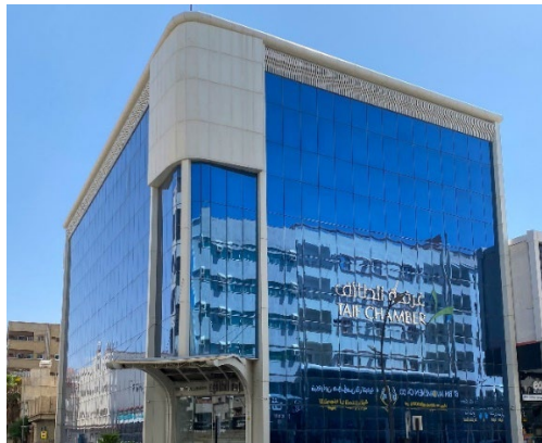
Figure (11): Depicts the Taif Chamber of Commerce building, with its facades covered with curtain wall.
