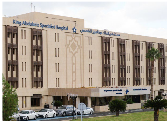
Figure (2) shows a picture of King Abdulaziz Hospital, whose facades were covered with natural marble.
