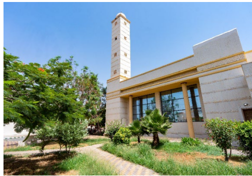
Figure (6): illustrates a picture of the Taif University Mosque, whose facades were covered with limestone.
