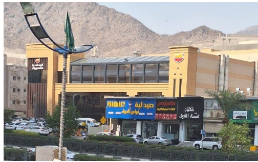
Figure (5): illustrates the cladding of facades with Hashemite stone.
