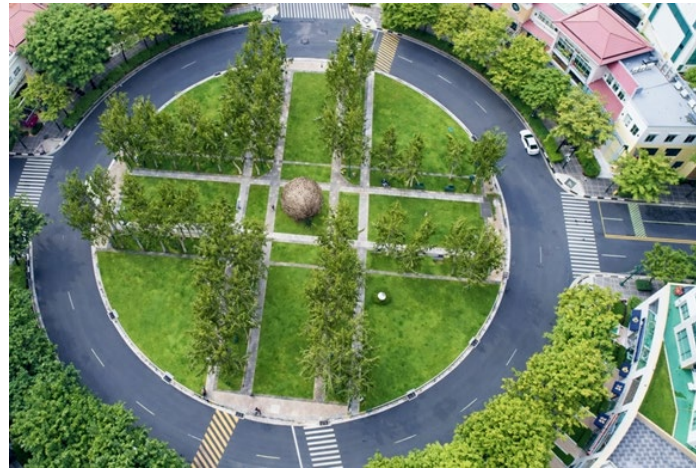
Figure 3. Burgos Circle, BGC, Philippines, “Flood Control Tunnel” (Aerial View) [33]
